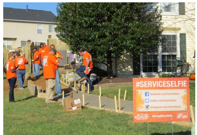
The concrete rear access ramp under construction.
